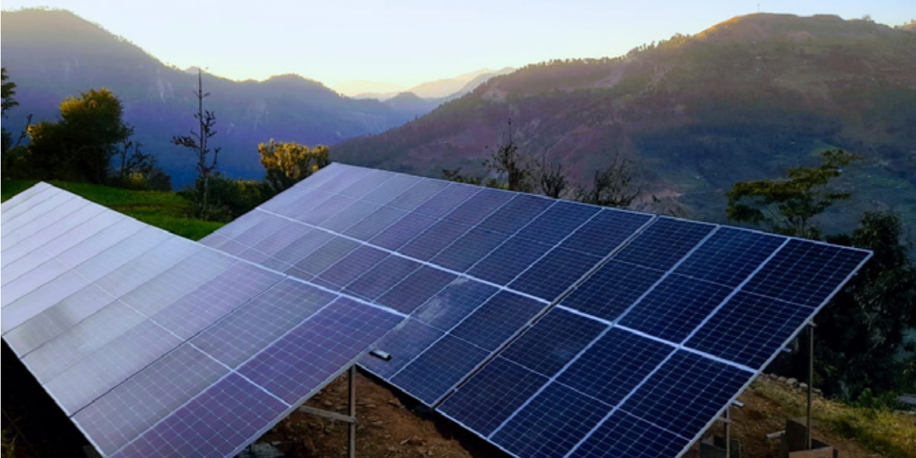
Establishment of solar-based lift irrigation system in Pali village of Dullu Municipality in Dailekh. Photo: LI-BIRD Photo Bank
