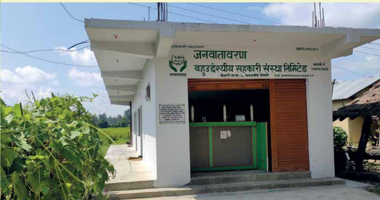
Newly built service building with seed storage of the Janawatawaran Multipurpose Cooperative, Kailali. Photo: Niranjana Pudasaini, LI-BIRD
